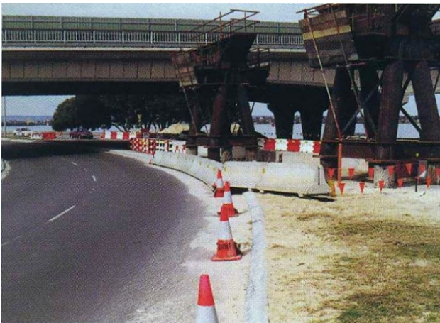
Figure 3.3: Example road work site treatment – barrier location
